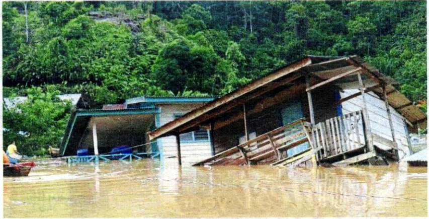
Badly damaged: Several houses that were toppled in Long Busang due to the sudden floods.
